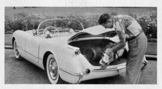
THE SLEEK REAR DECK of the Corvette conceals a generous luggage compartment—far more spacious than most sports cars. The spare tire is in a well under the floor, and the radio antenna is built into the deck lid.
